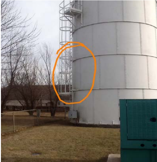
Access to Tanks
