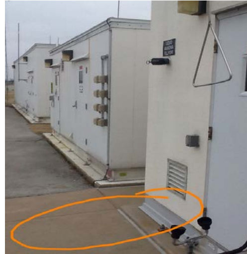
No Spill Containment During Delivery
