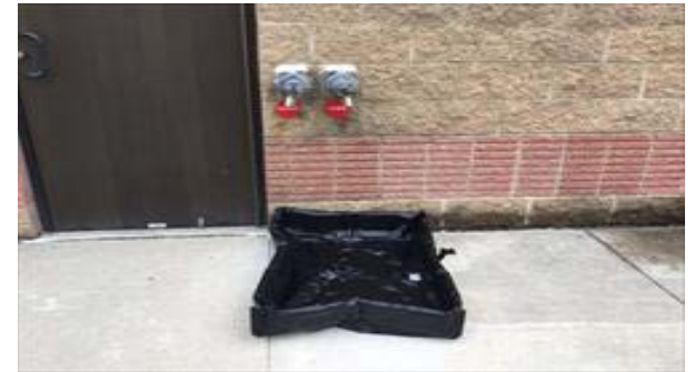
Portable Spill Containment for Deliveries
