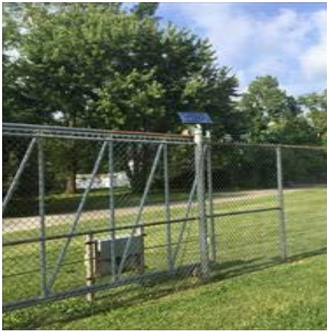
Solar Powered Gate Operation
