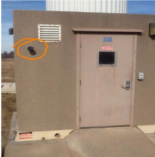
Unlabeled and Unsecured Fill Points
