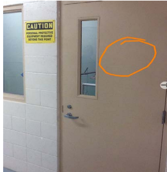
No Hazard Signage on Chemical Room
