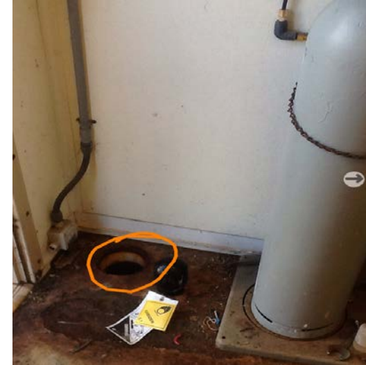
“Mystery” Floor Drain in Chlorine Room
