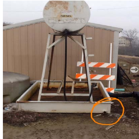
Inadequate Containment
