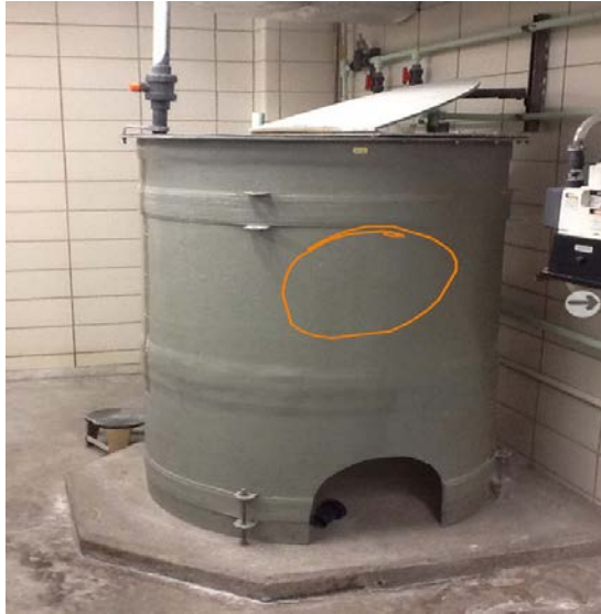
No Identification on Chemical Tank
