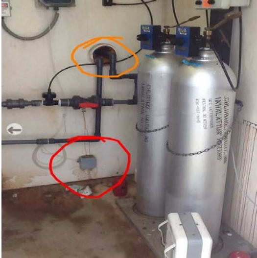
Air Leaks to Other Rooms; Not Checking Sensors
